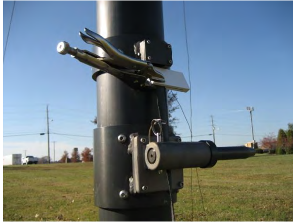
Figure 8-3 Once Load has Been Fully Transferred to the Clamp Block, Winch can be Removed
