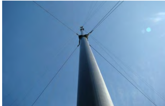
Figure 4-29 When Guy Lines are Being Tensioned, Stand at Base of Mast and Site Mast for Vertical
