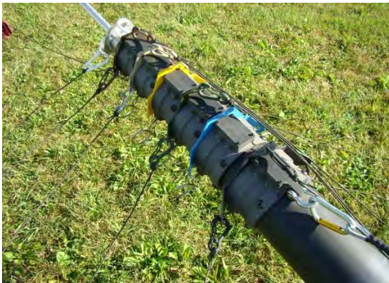
Figure 4-16 Attach Remaining Guy Lines
