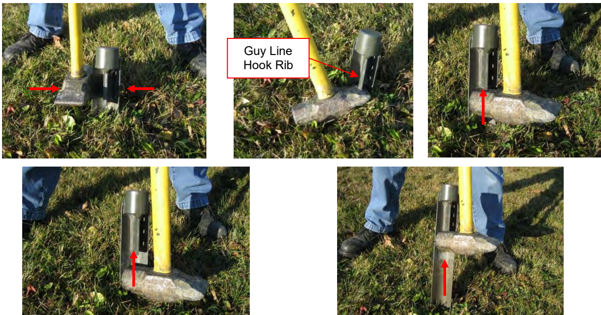
Figure 5-12 Hit Each Guy Stake on Each Edge and Use Hammer to Pry Under the Guy Line Hook Rib
