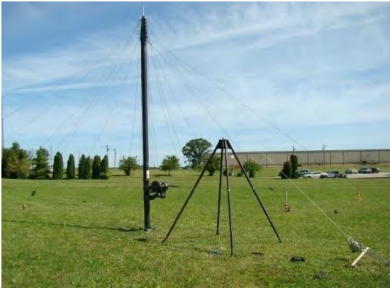
Figure 4-18 Raise Mast to Vertical
