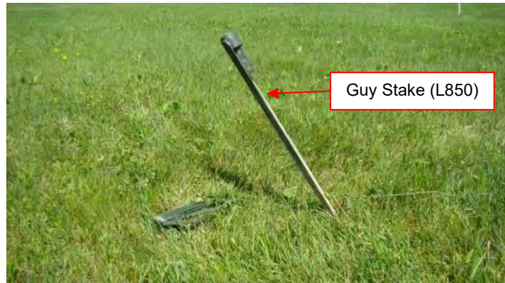
Figure 4-4 Hammer Guy Stakes at 60° Angle at Each Loop of Radius Rope
